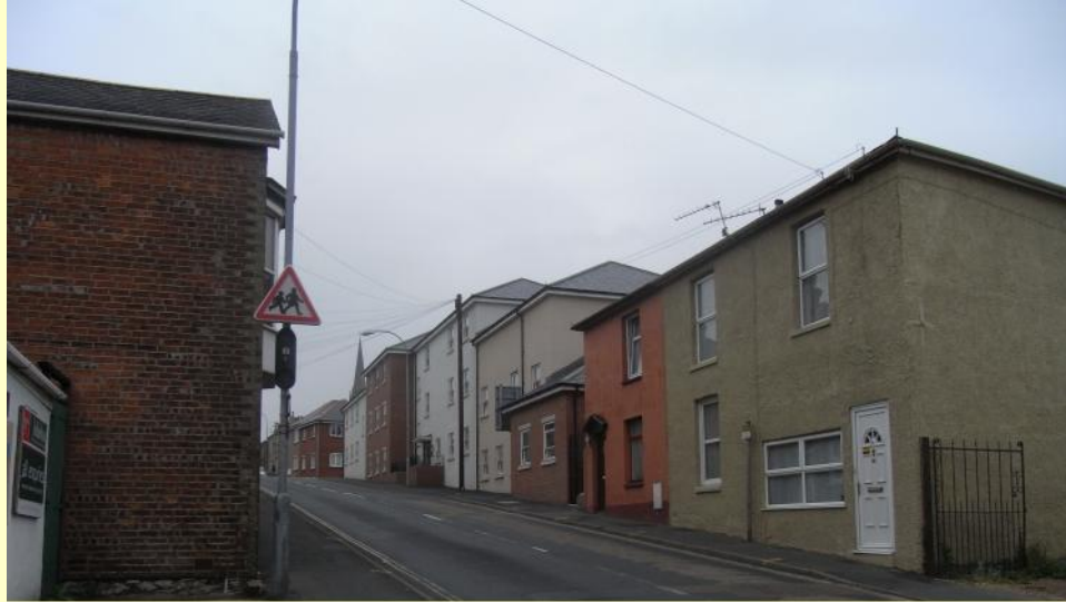
The Steam Mill was roughly where the red brick building between the two white ones is situated
